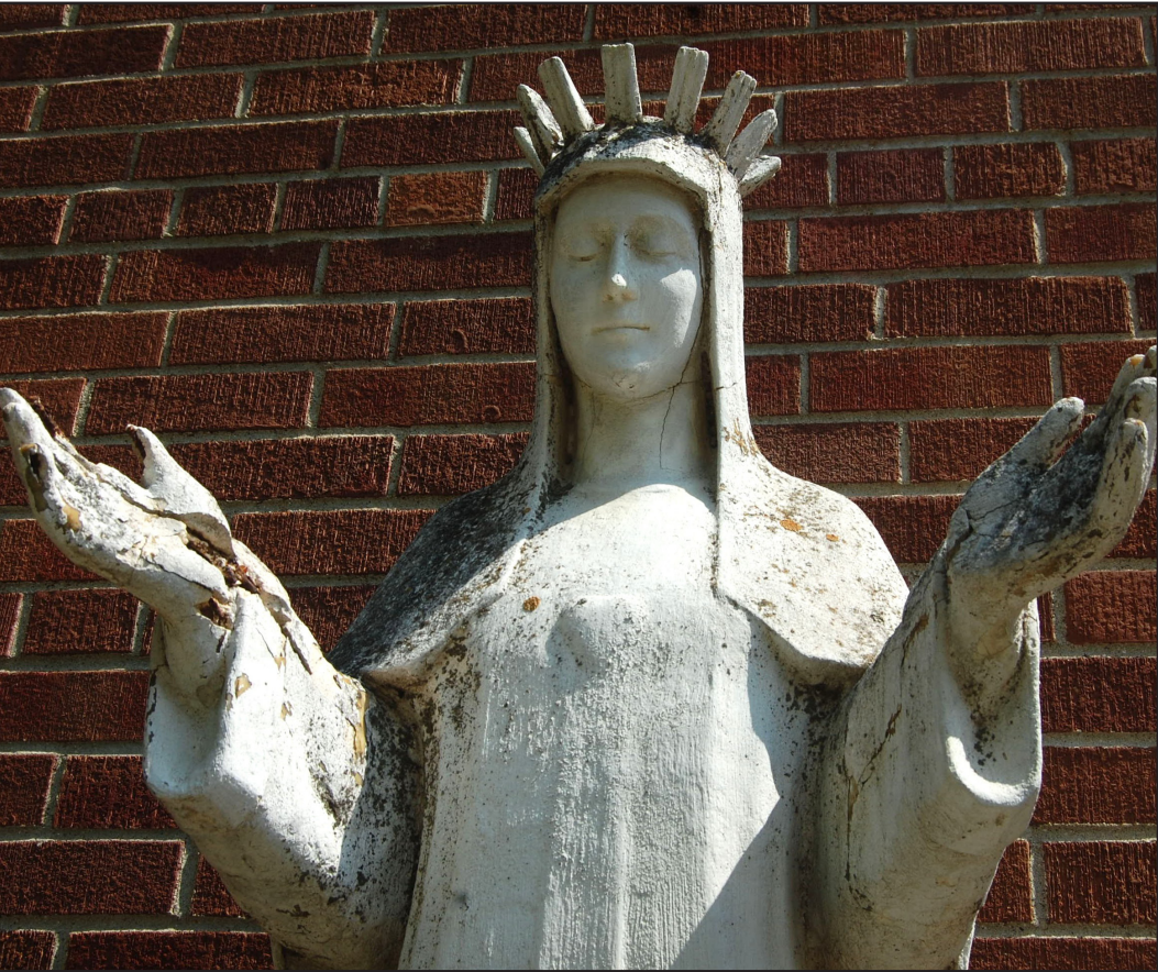
The Our Lady of Beauraing statue outside St. Edward’s Catholic School has cracks in several places and the hands and wrists are deteriorating. Mascot photo by Scott Thoma
